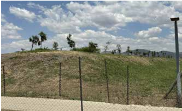
Trees were recently relocated and planted along PCD to construct a mitigation measure berm
