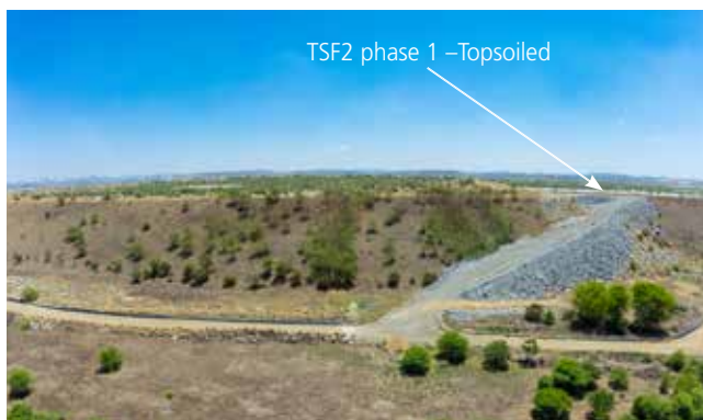
TSF 2 phase 1 – Topsoil and revegetation in progress
