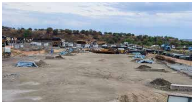
Ongoing construction at mining engineering workshops
