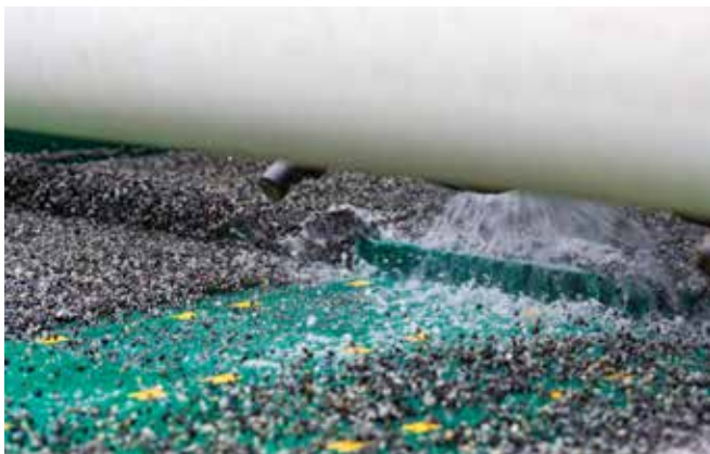
Upgraded sewerage treatment plant
