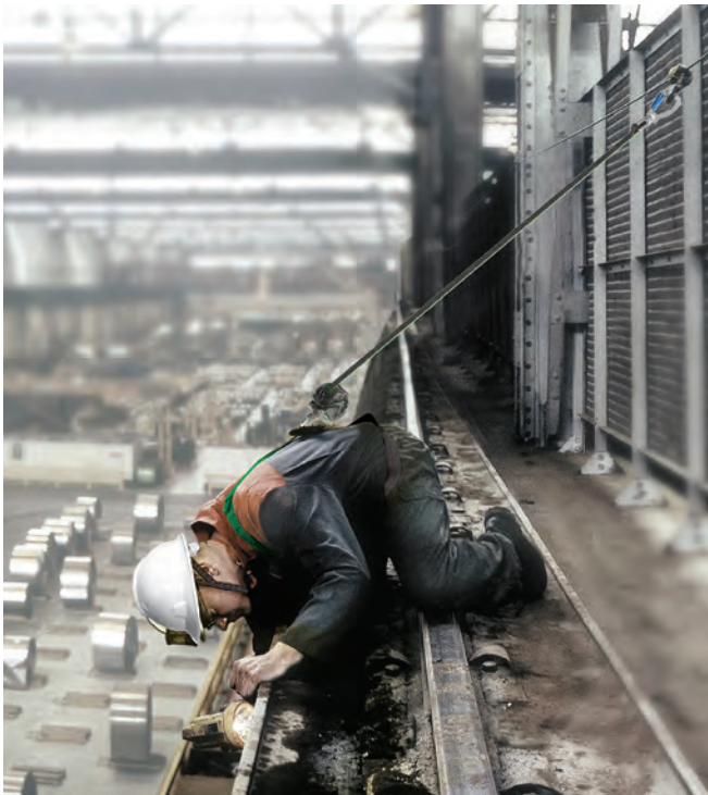
Lloyd's on-site training
