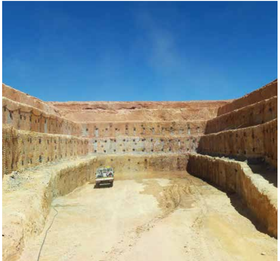
Completed box-cut for shaft collar civils.
