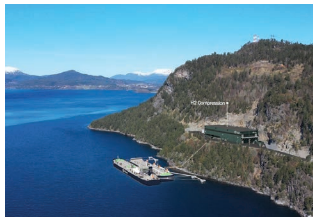
Figure 2 Compression plant located at adjacent site to a dedicated jetty for bulk export using Provaris H2Leo storage barge and H2Neo carrier
