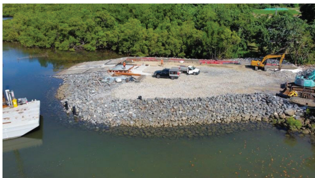
Newell Beach boat ramp newly built with Mt Carbine's green waste rock.
